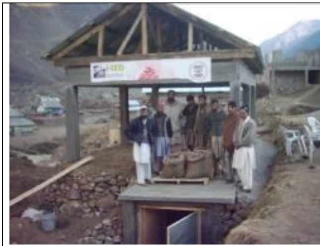
Photo 2 Example of Potato Storage Building and Diagram of Chimney Construction
